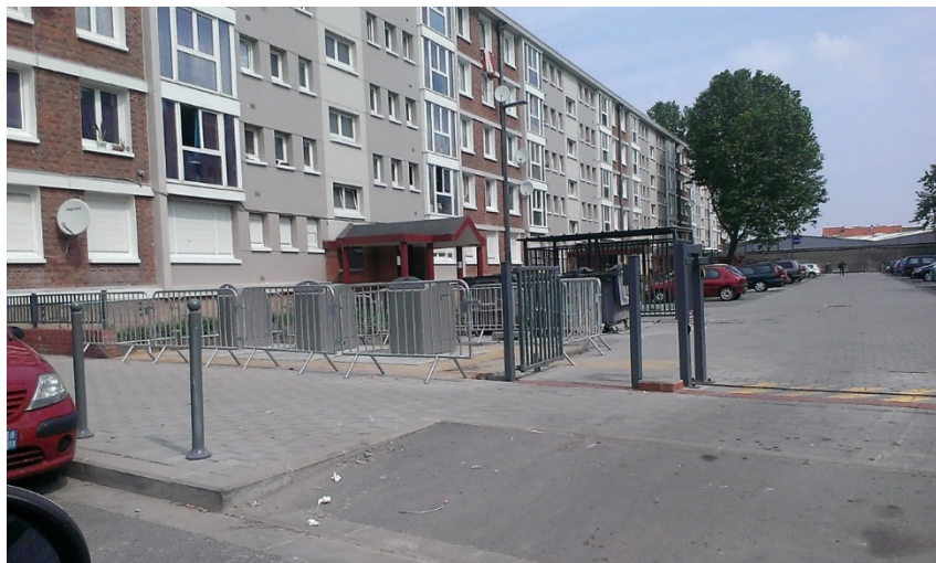
Figure 21: Rehabilitation and external works in Lille Sud
