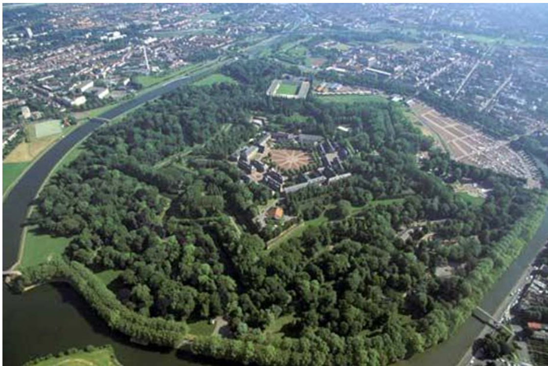
Figure 3: Vauban Citadel, central Lille
